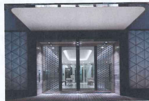
Queen's Apartments Stiff+Trevillion for Derwent London Contract value: £9m. GIA: 2729m 2
