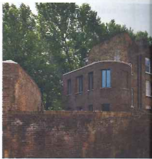
HULT International Business School Sergison Bates Architects for HULT Business School Contract value: £3.7m. GIA: 4300m 2
